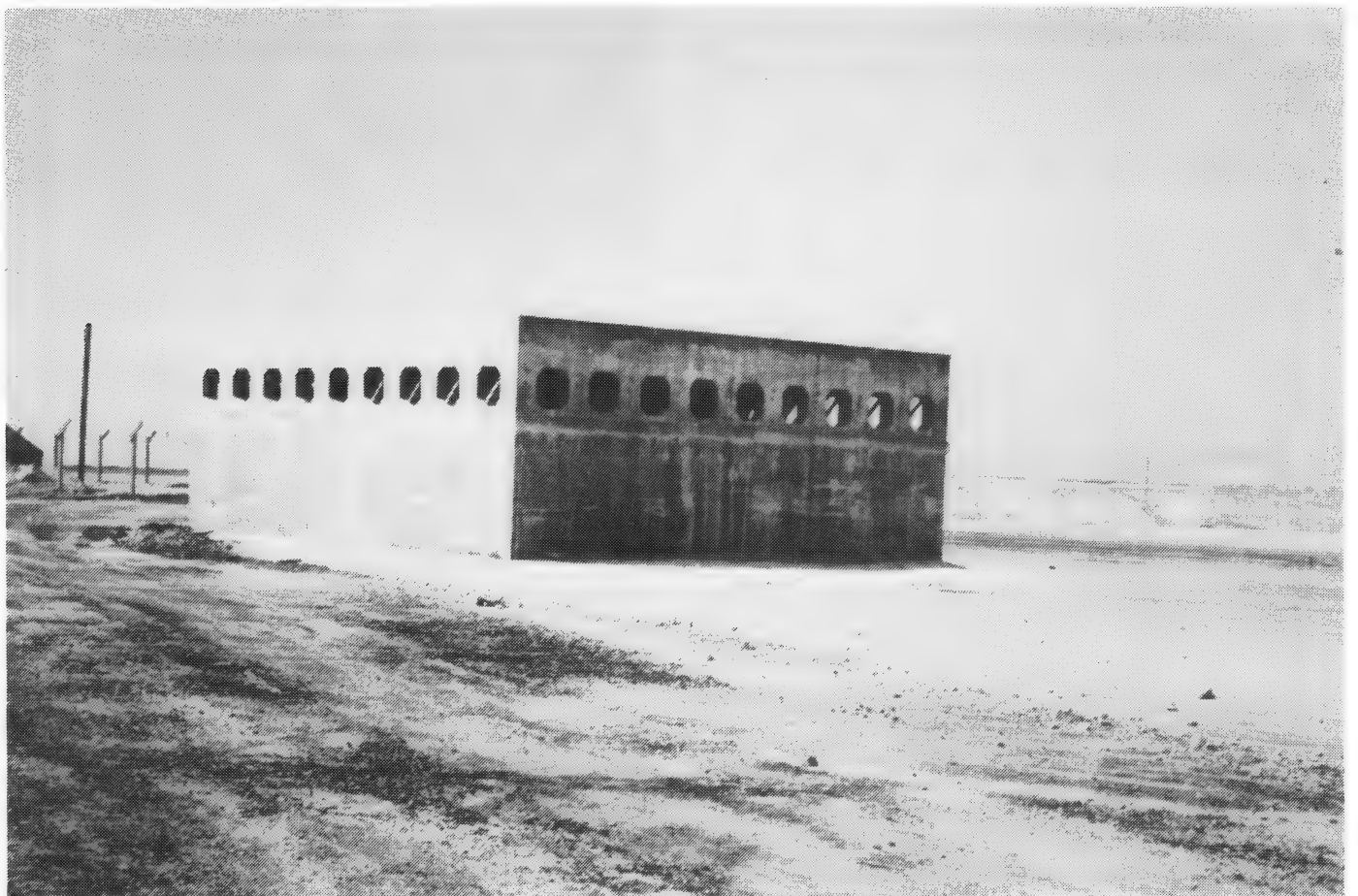
FIGURE 4-11. ONE OF THE NAVY BUILDINGS, ENGEBI
